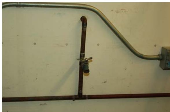
Figure 7. MACC's water pipe and hose bib.
