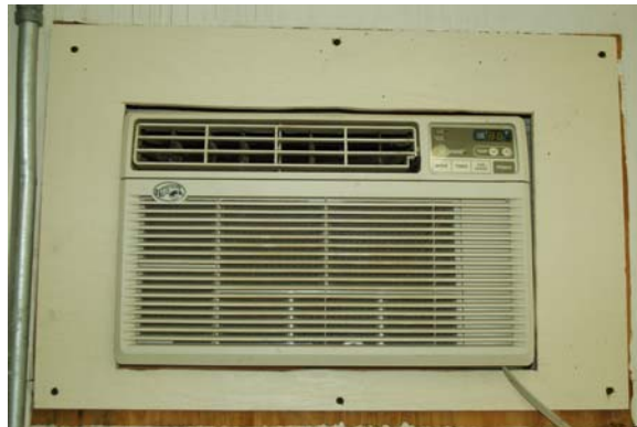
Figure 9. A standard household window A/C unit was installed in the wall of each container.
