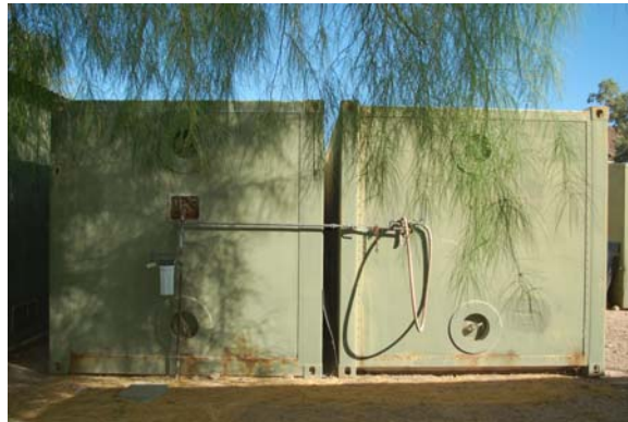
Figure 3. Back view of the MACC shows where water is plumbed into both buildings via pipe.
