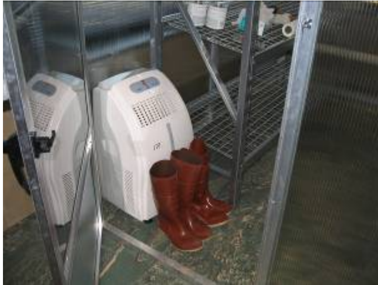
Figure 4. The portable heating/air condition unit and dedicated footwear placed in each room.
