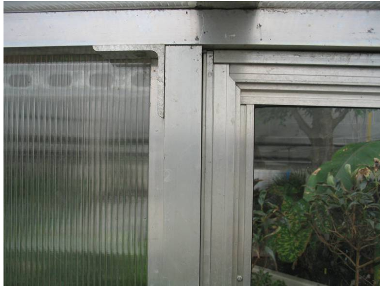
Figure 3. Close-up of the 1inch (2 cm) aluminum angle pieces holding the 1.5 x 1.5 inch (3.8 x 3.8 cm) aluminum tubing and storm door.
