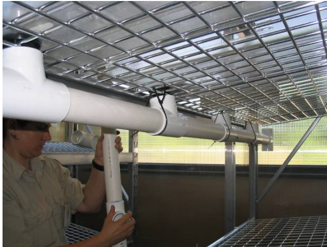
Figure 6. The over-sized drain system under each shelf being installed in the IAR.
